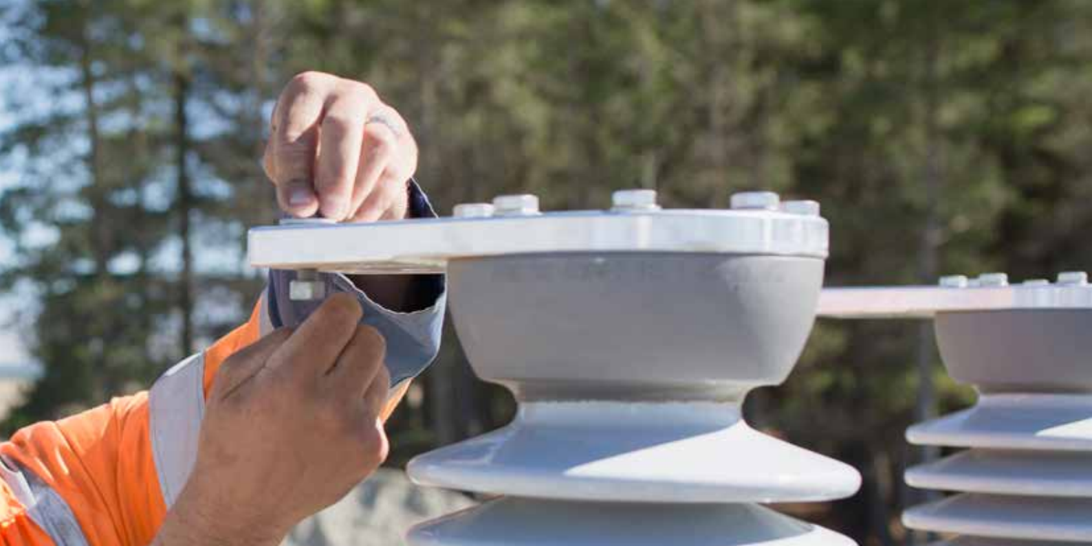
Construction of Lindis Crossing substation
