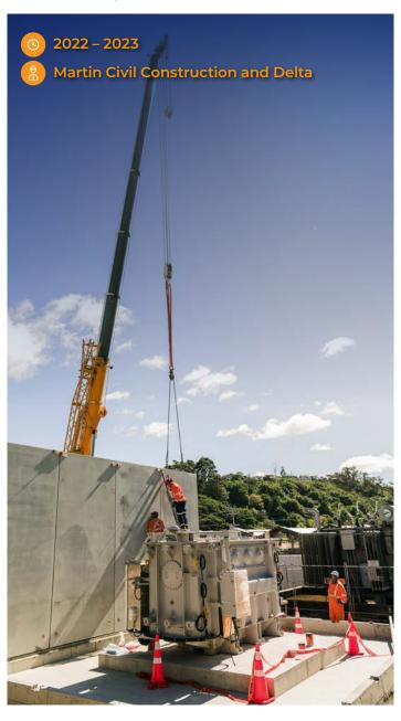
Work is progressing well with the \$8.4m upgrade. We are replacing the existing aged equipment with new modern switchgear and transformers. We'd like to thank the local residents for their patience for any disruptions while we undertake this work.
