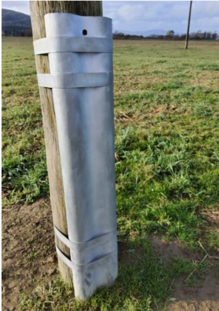
Figure 8.2: Example of a wood pole reinforcement
