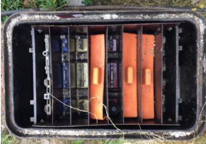
Figure 8.76: Decommissioned Henley underground link box
