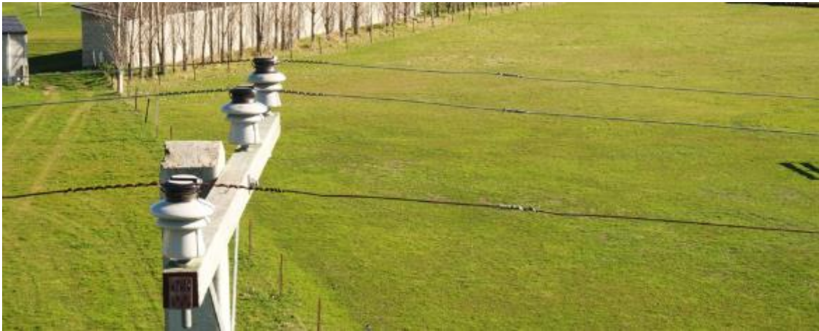
Figure 8.21: Rusty No. 8 wire at an insulated tie point due to bi-metallic corrosion
