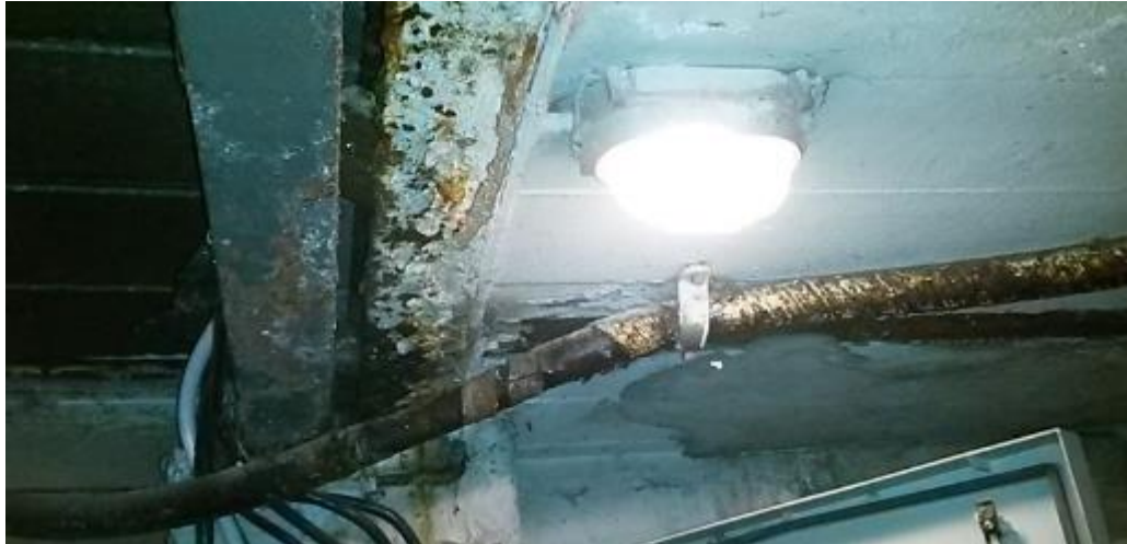
Figure 8.82: Example underground distribution substation condition
