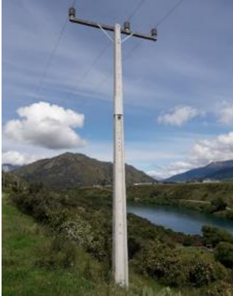
Figure 8.1: Example of a concrete pre-stressed pole
