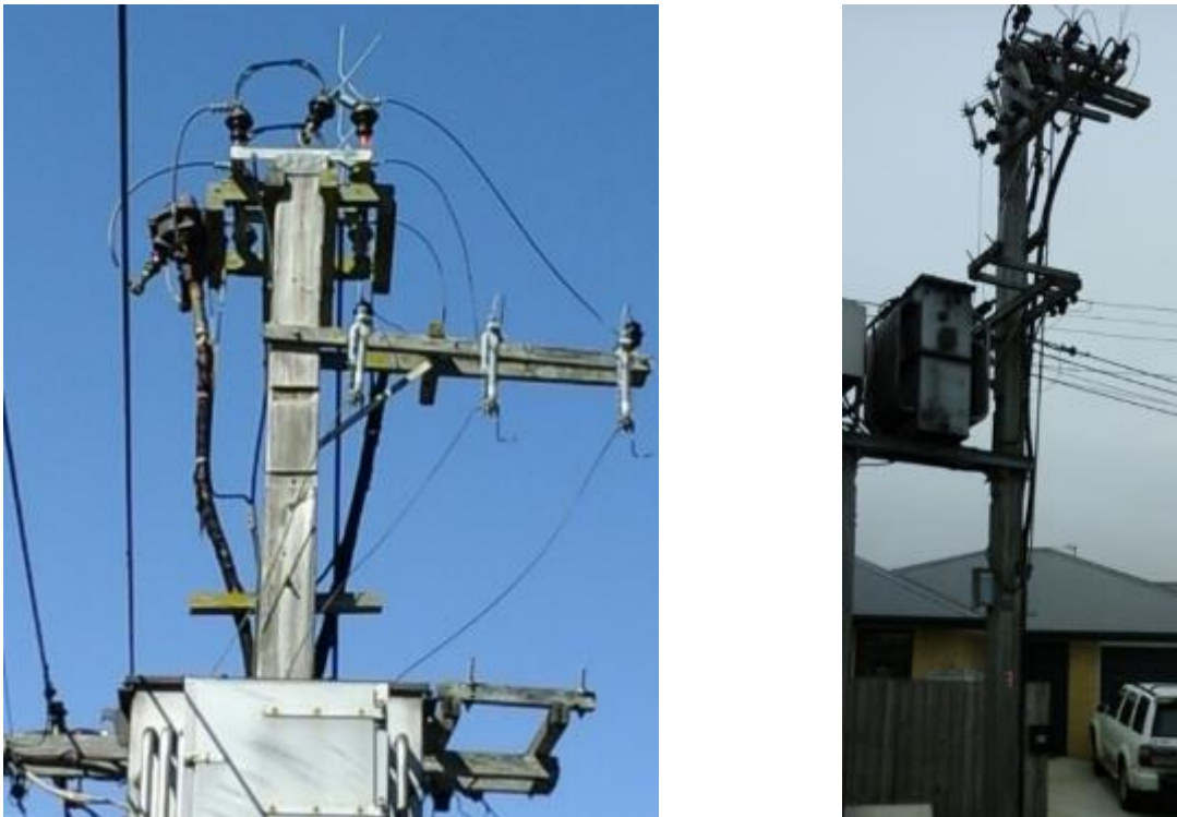
Figure 8.90: Legacy pole-and-a-half substation with an ABS and two cast iron pot head terminations
