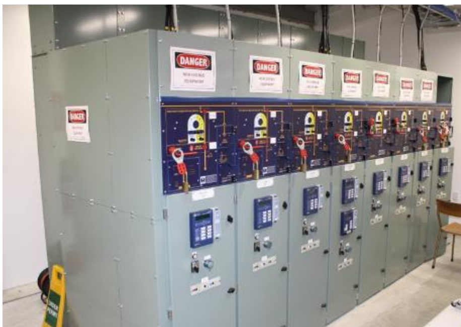
Figure 8.51: Modern vacuum interrupter indoor switchboard at Carisbrook zone substation
