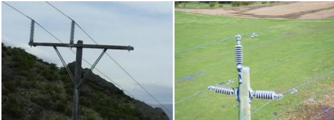
Figure 8.15: Floating conductor following mechanical insulator failure (left) and re-configured to delta construction with Stockbridge dampers fitted (right) 14
