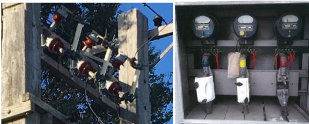
Figure 8.67: EETEE HRC fuses (left), and 'homemade' aluminium box containing LV JW fuses and MDIs (right)
