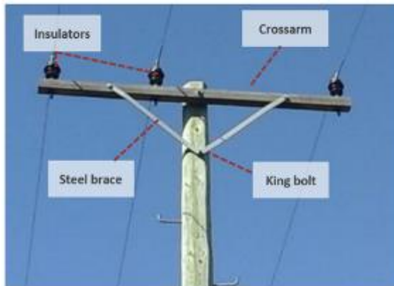
Figure 8.8: Typical crossarm arrangement
