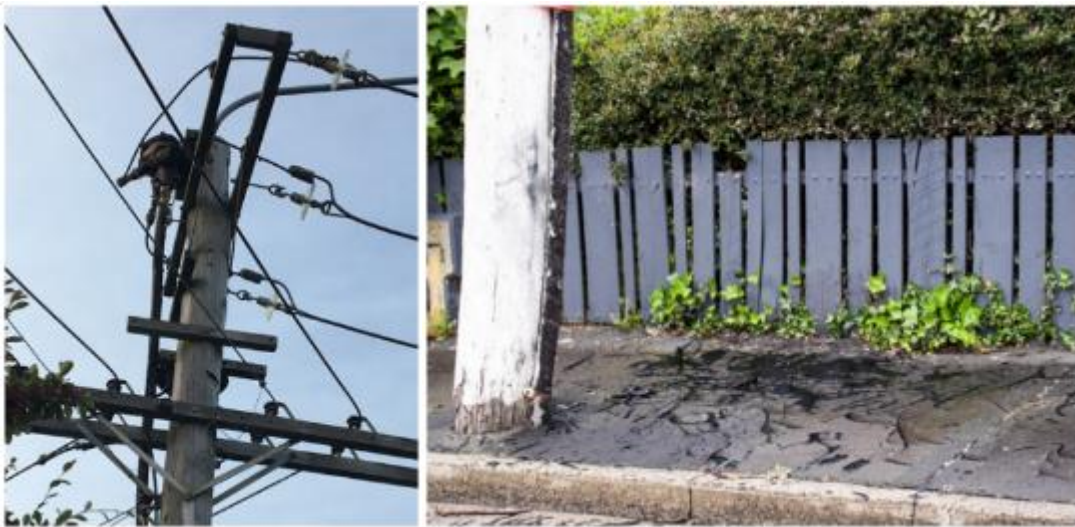
Figure 8.36: Cast iron cable termination (left) and bitumen sprayed after cast iron cable termination failure
