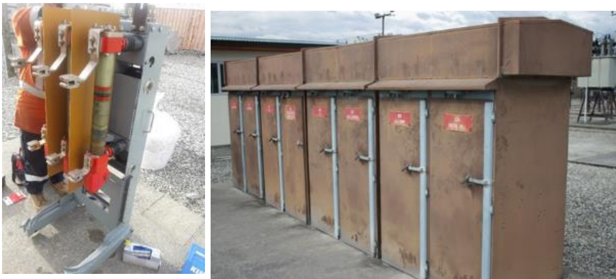
Figure 8.57: Indoor minimum oil-filled circuit breakers (left) installed in outdoor cubicles (right)
