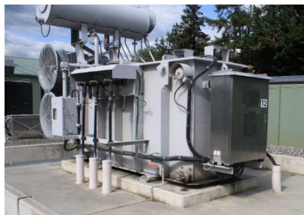
Figure 11-29: Power transformer
