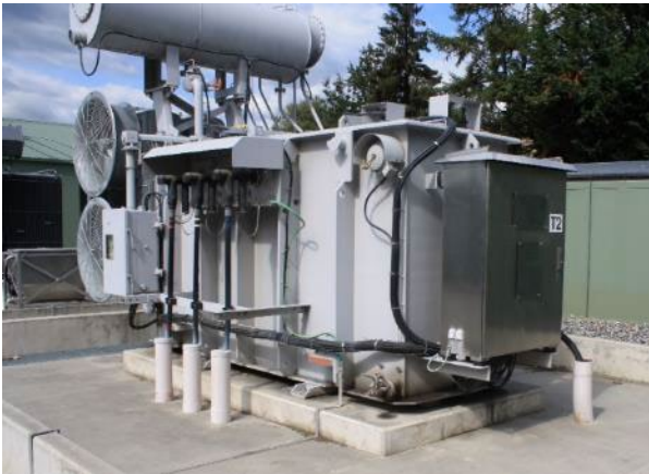
Figure 11-31: Power transformer
